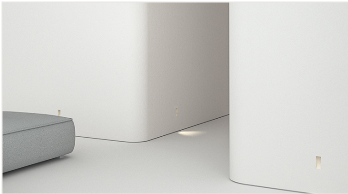
Plaster wall, painted to match — the aperture disappears by day.
